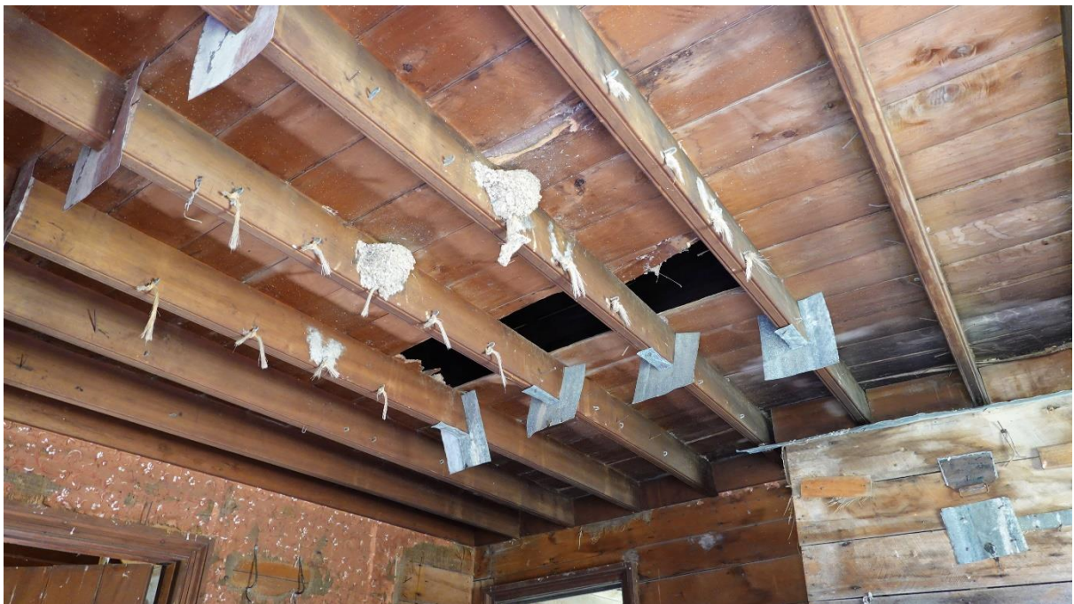
Figure 27. Nineteenth century cottage, detail of construction. Note hand-planed rafters.
