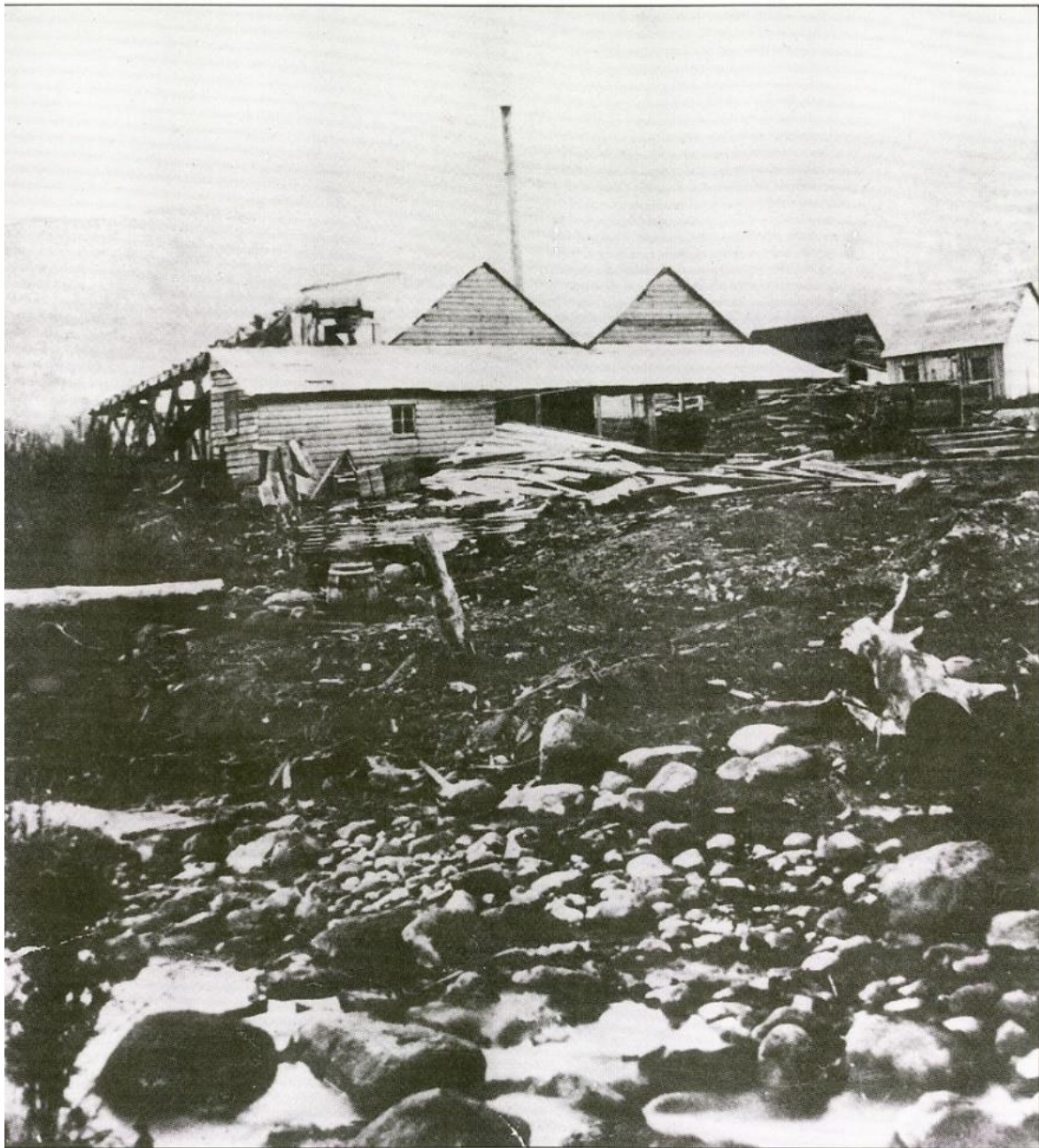
Figure 11. Saxon and Williams' Robinson Bay Steam Sawmills, known locally as the Matlock Mill, operated from 1865-c.1877. Flume and waterwheel upper left; blacksmith shop right. (Ogilvie 1990:169)
