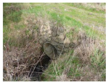
Figure 28. Stone rubble and concrete culvert (14) along access track (8) (N. Cable 21/07/2021).
