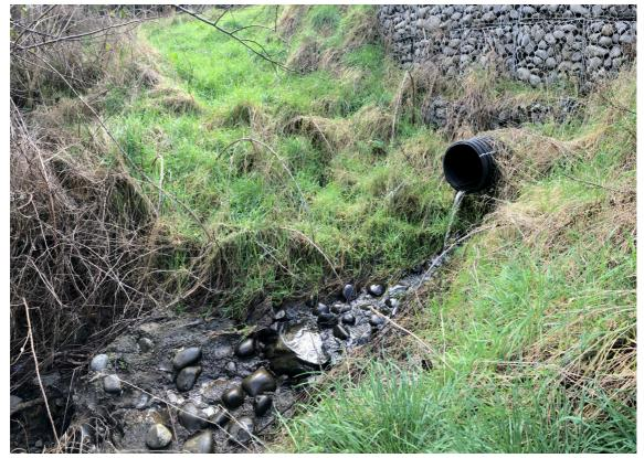
Looking upstream at the culvert outlet pipe in the road to the Akaroa Cottages. There is a vertical drop of 0.65 m from the pipe outlet, and a second smaller vertical drop downstream of the concrete sill where the stream channel has eroded away (just out of the image).
