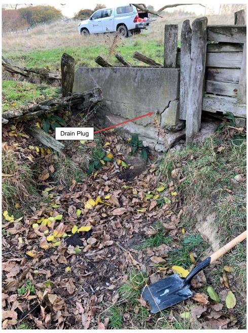
Figure 10: Man-made channel extending from below the northwest end of the sheep dip down to the terrace shown in Figure 8. Notice drain plug in the side of the dip.
