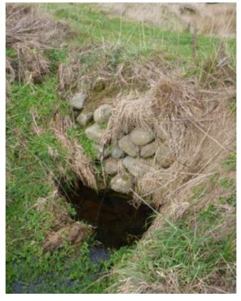
Figure 29. Second stone rubble and concrete culvert (15), partially submerged, under access track (8) (N. Cable 21/07/2021).
