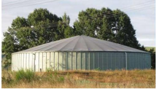
Figure 2. Example of 'Kliptank' storage with cover (Dimensions unknown)
