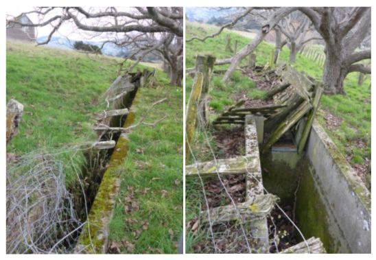
Figure 36. Cement-rendered brick sheep dip, located along fenceline above stream flat (N. Cable 21/07/2021).
