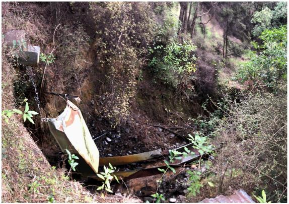
Looking downstream at a degraded metal ramp from the road culvert under SH75. The vertical drop is at least 2m
