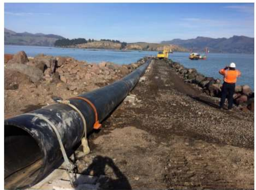
Photograph 1: Launch of Governor Bay Submarine Pipeline
